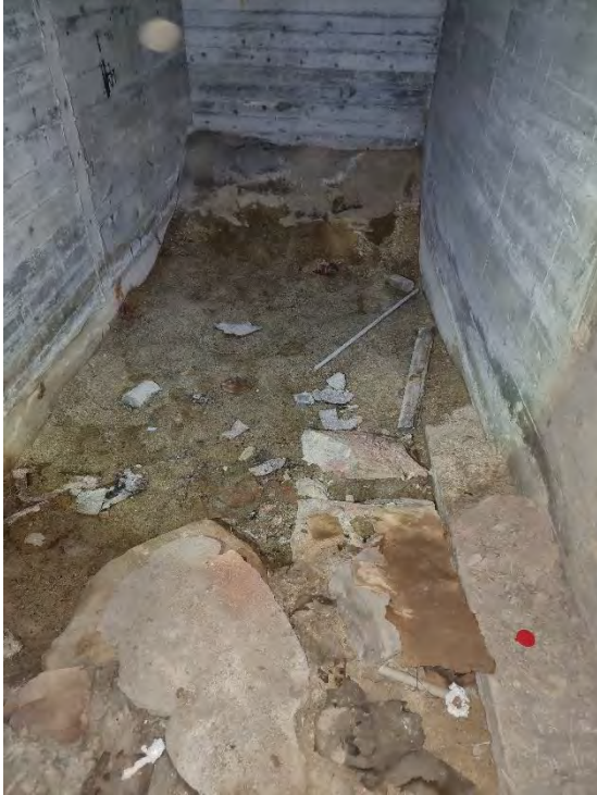
Figur 45 Krypgrund under Storkök
