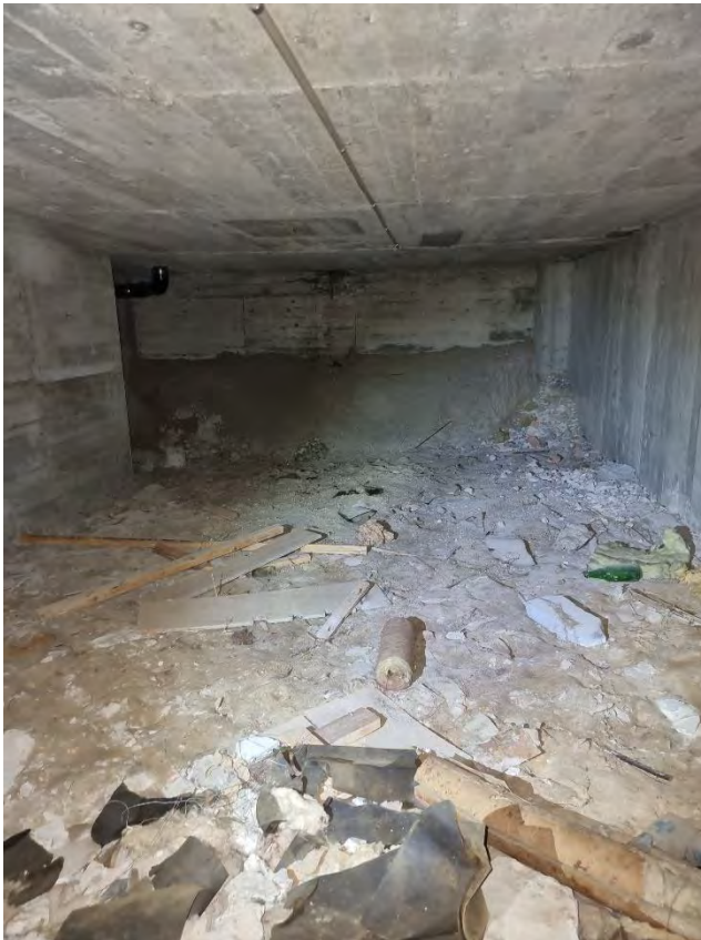
Figur 47 Krypgrund under Storkök
