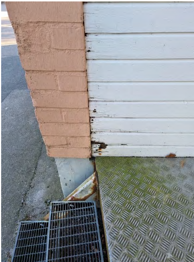
Figur 16 Skadad panel
