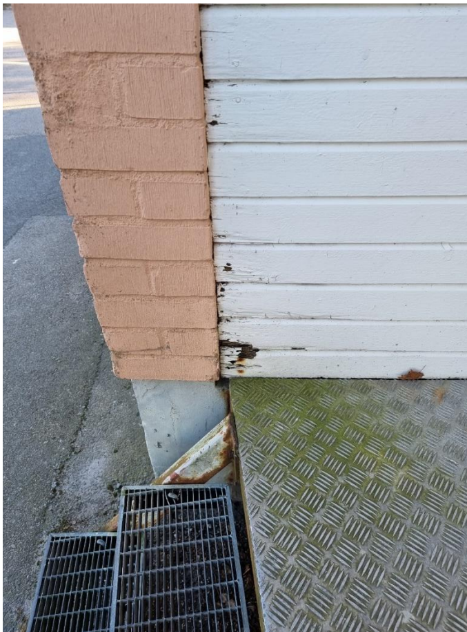
Figur 16 Skadad panel
