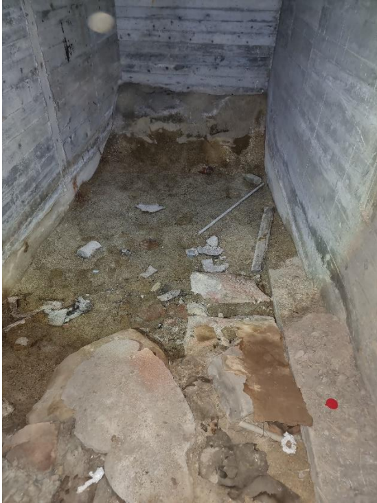
Figur 45 Krypgrund under Storkök
