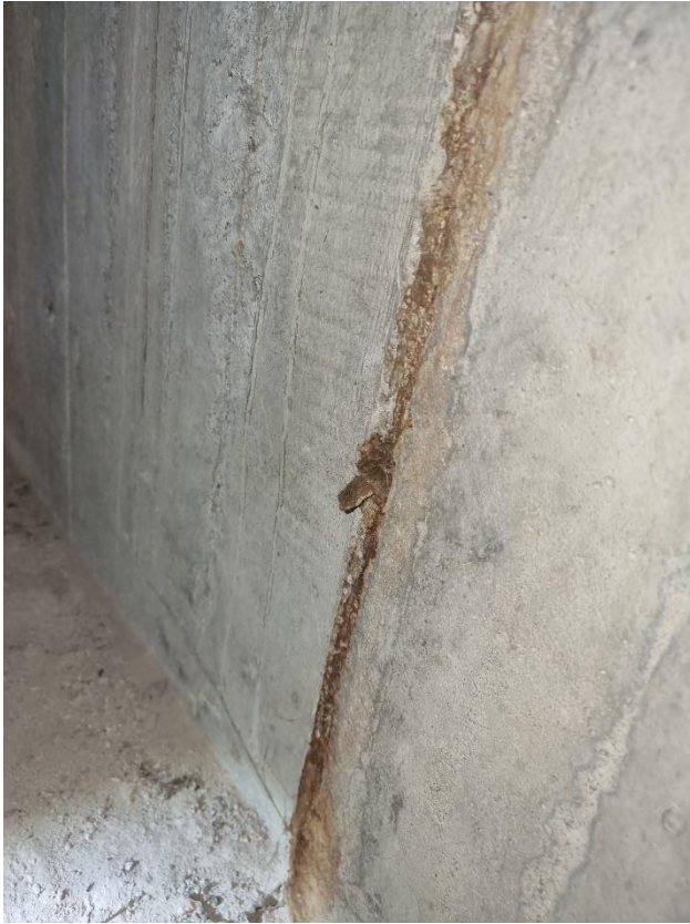
Figur 48 gjutfog asfboard
