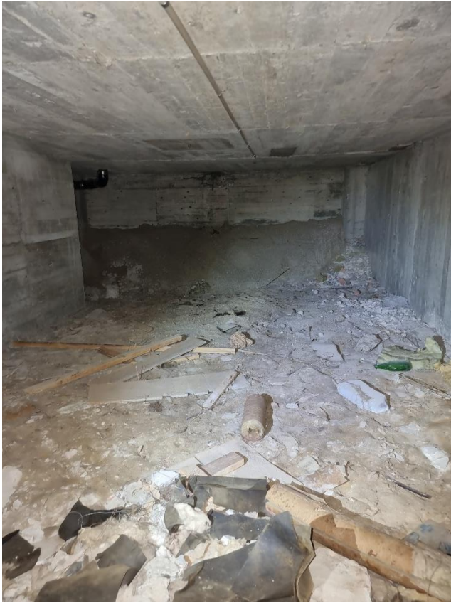
Figur 47 Krypgrund under Storkök
